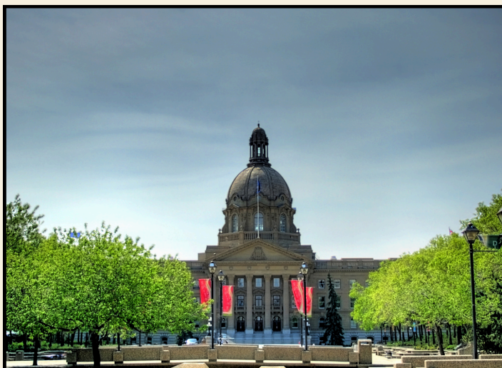
The Alberta Legislature Building, completed in 1913. Photo: WinterE229, CC0.
